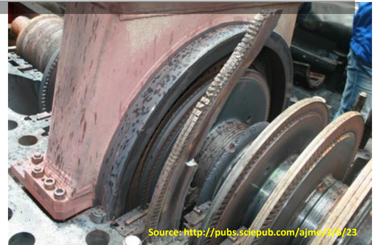
Fig. Damaged Steam Turbine Disk
